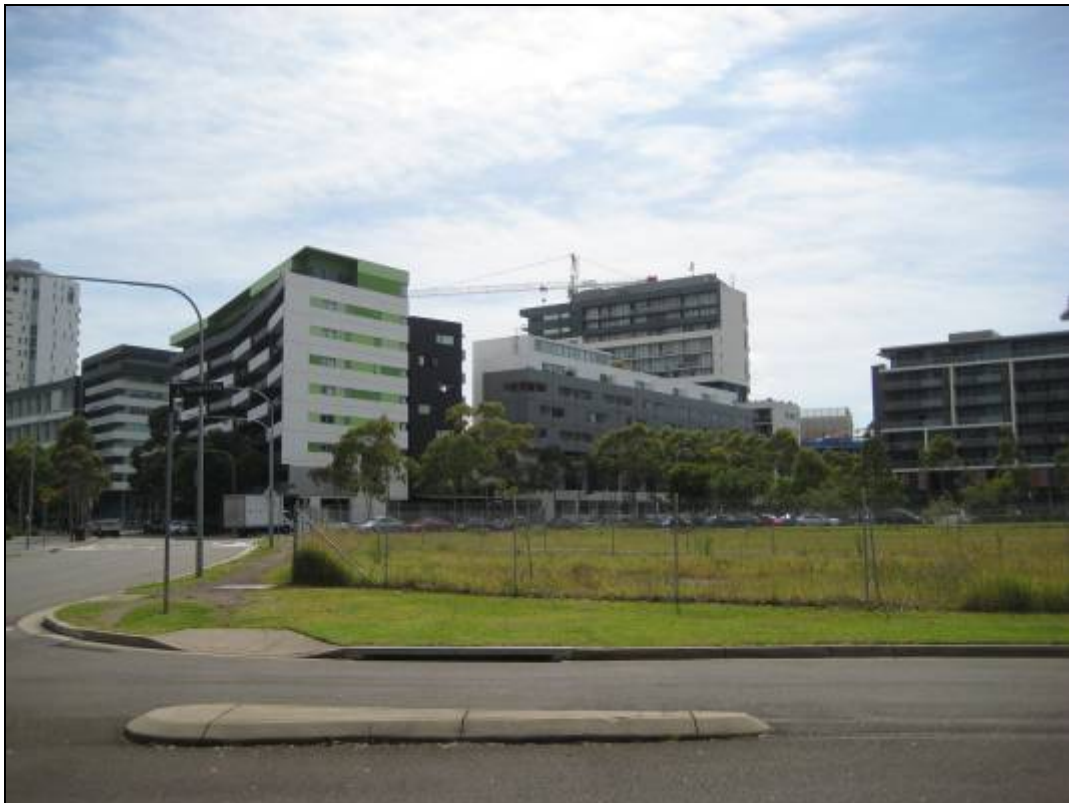
Figure 6 - The 'Form' development located to the north of the site fronting Gadigal Avenue and Hutchinson Walk
