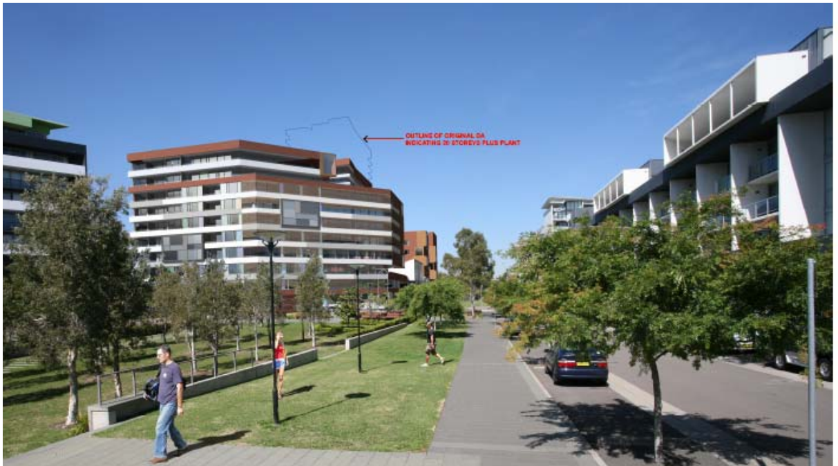
Figure 12 - Photomontage of the northern elevation of the approved development as viewed from Joynton Park
